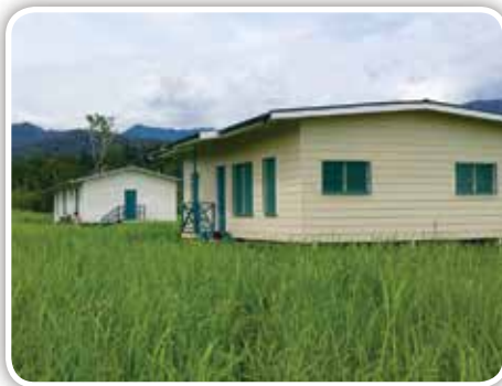
Above: The Buhalu Medical Clinic and staff house in Papua New Guinea were made possible in part through the Thirteenth Sabbath Offering.
