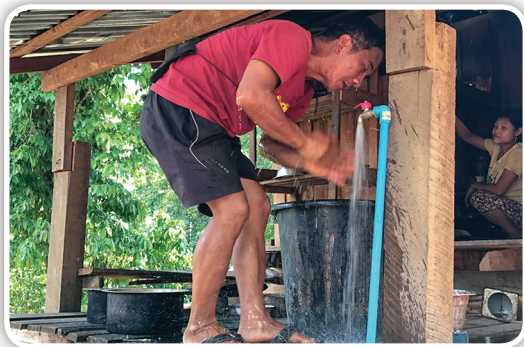
A villager using a faucet at the end of the new water pipeline.
